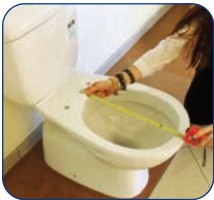
Measure from the centre of the bolt holes to the front of the bowl. (D)
