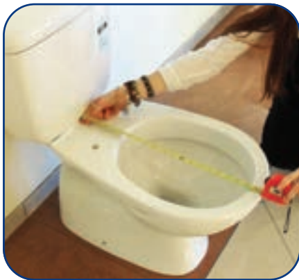
First thing to do is to measure from the front of the cistern to the front of the bowl. (A)
