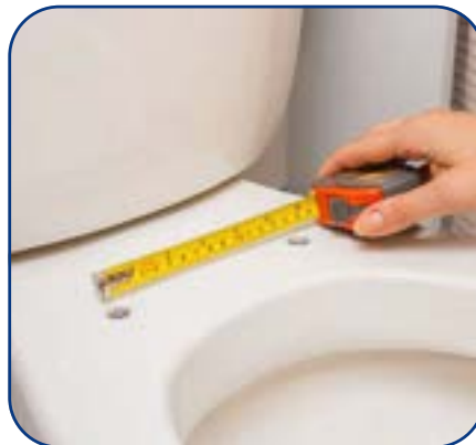
Measure the distance between the bolt holes (B)
